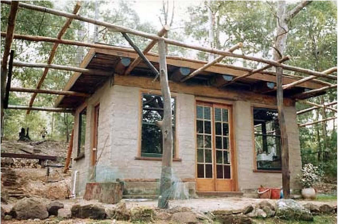
The new cabin. It had a sod roof.
